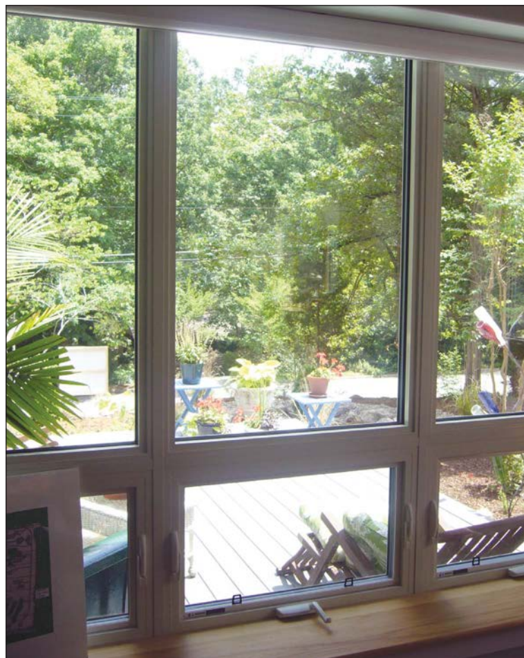
Triple-pane, argon-filled windows take up about 100 square feet of the south-facing wall.
