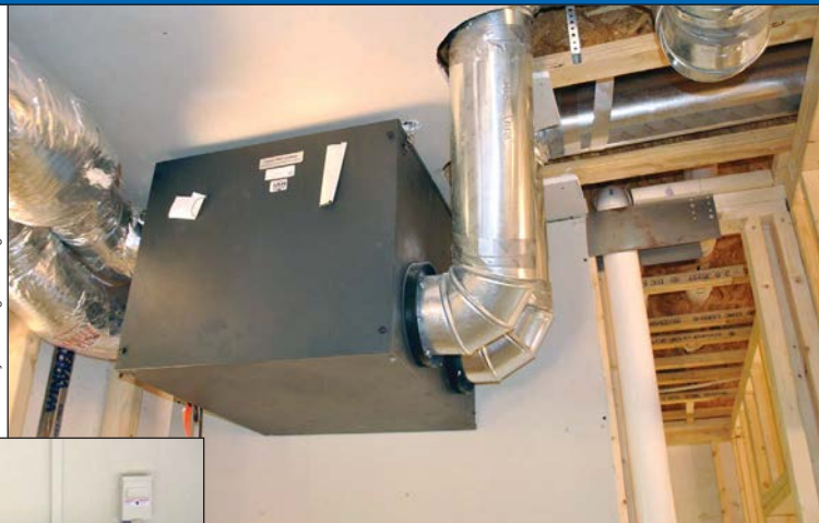
Above: An air-to-air heat exchanger exhausts stale air and brings in fresh air, but keeps about 75% of the heat while doing so.
